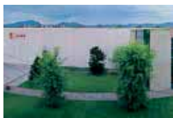
The New Factory
